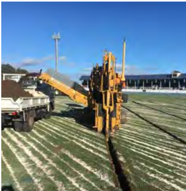
Installing sand slit drains into existing sportsfield
