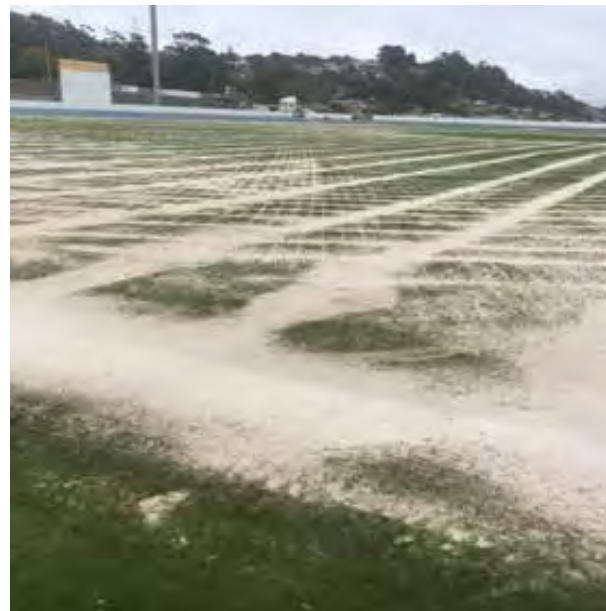
Installing sand slit drains into existing sportsfield
