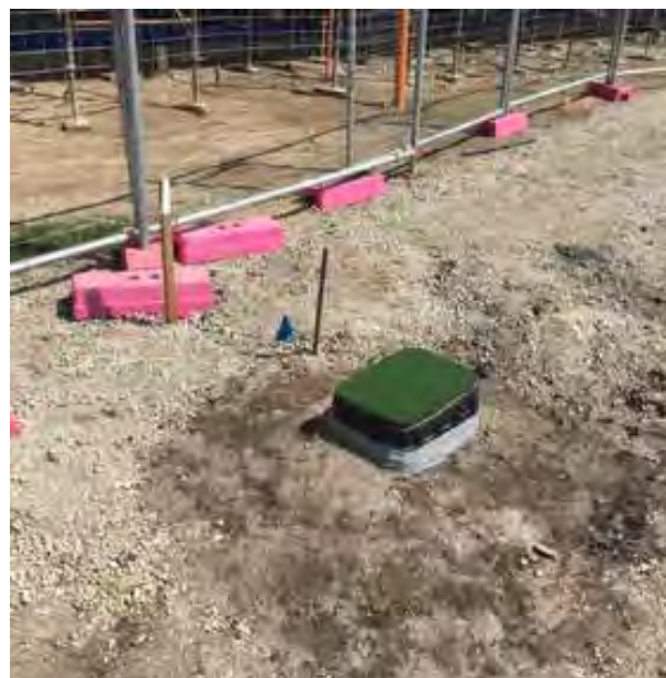
Installed solenoid box
