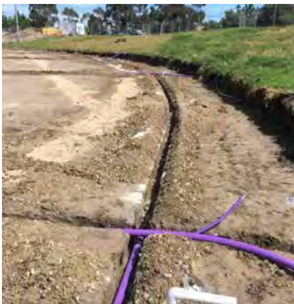
Installation of irrigation pipework
