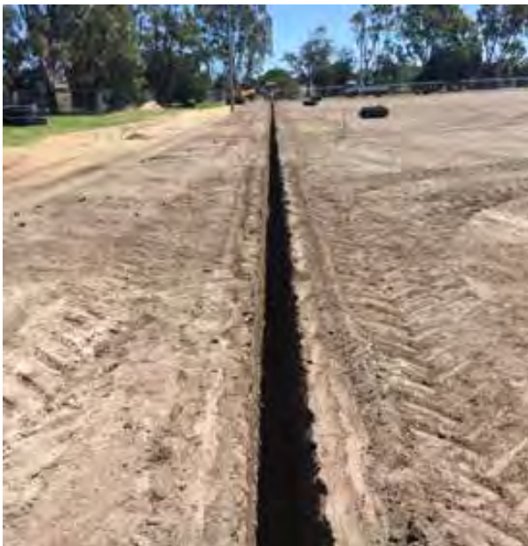
Trench dug prior to installing drain
