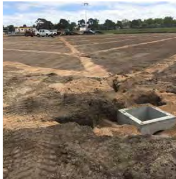
Subsurface drainage being installed in oval
