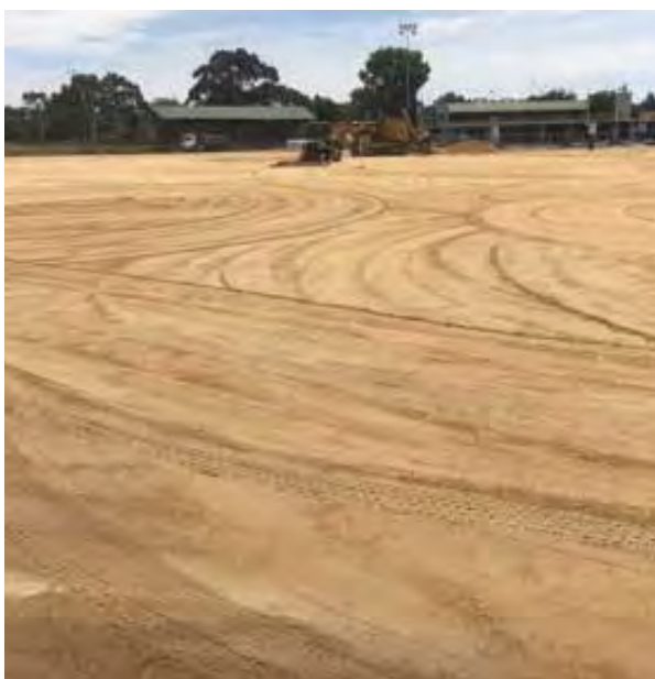
Installation of sand root zone layer
