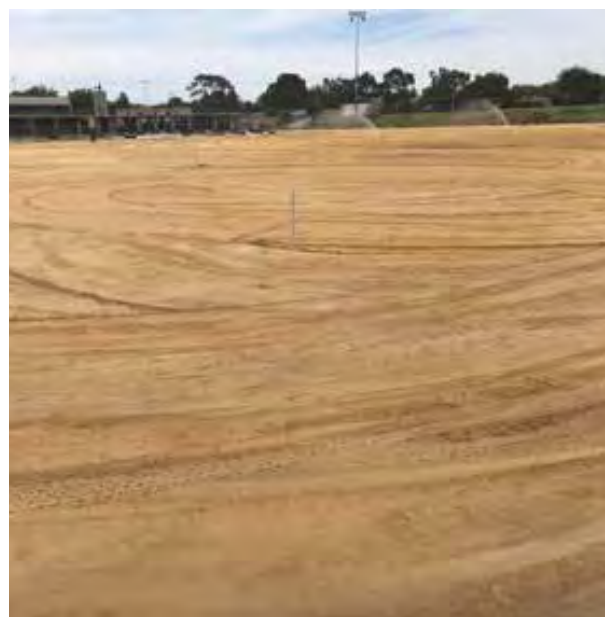
Installation of sand root zone layer
